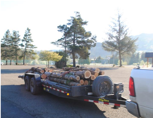
Log rafts were assembled offsite. The 10 rafts were 8 to 10 feet in length and compact enough to fit on a single trailer.
